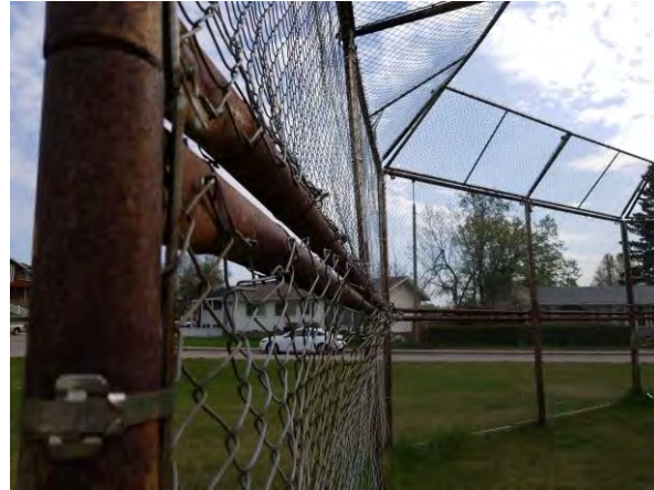
Rusting and damaged baseball backstop fencing at Erith Park off Macleod Avenue in the Central District
