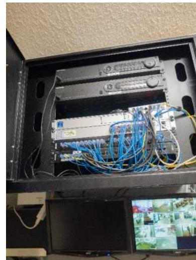
In the pro shop, a Bogen TPU35B Mixer-Amplifier, used for an intercom system, is installed behind the television. Network cables run through this device but it's not clear if its functional. It is Associated's understanding that the intercom system is not in use.
