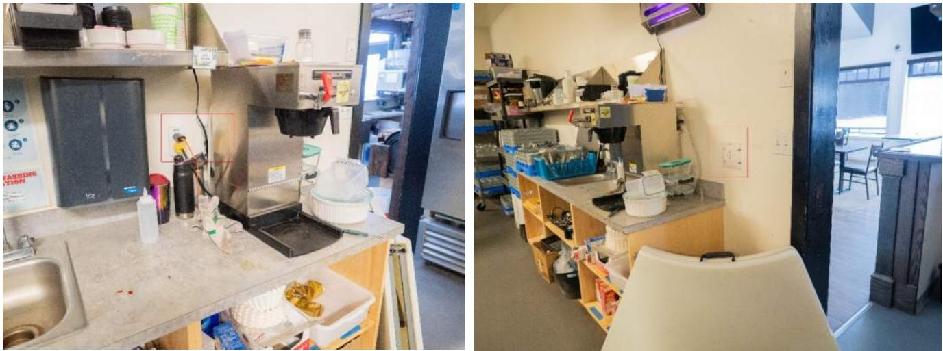
Receptacles mounted as part of the stainless-steel sink system appear to be part of a kitchen multi-outlet assembly, but confirmation that they are protected by Class A ground fault circuit interrupters was not seen. To meet the current
