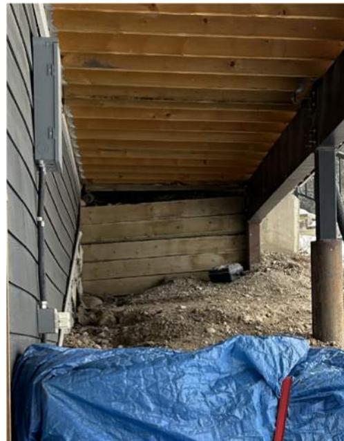
**Photo 10: South Side, Sloughing Around Retaining Structure to be Monitored**
