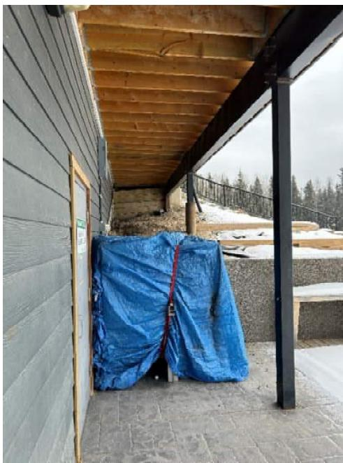
**Photo 9: Exterior Balcony – South Side, Sloughing Around Retaining Structure**
