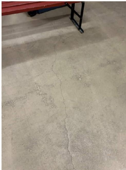
Photo 1: Slab-on-grade, Minor Cracking
