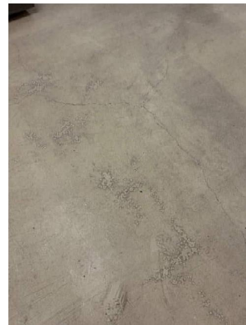
Photo 2: Slab-on-grade, Minor Cracking
