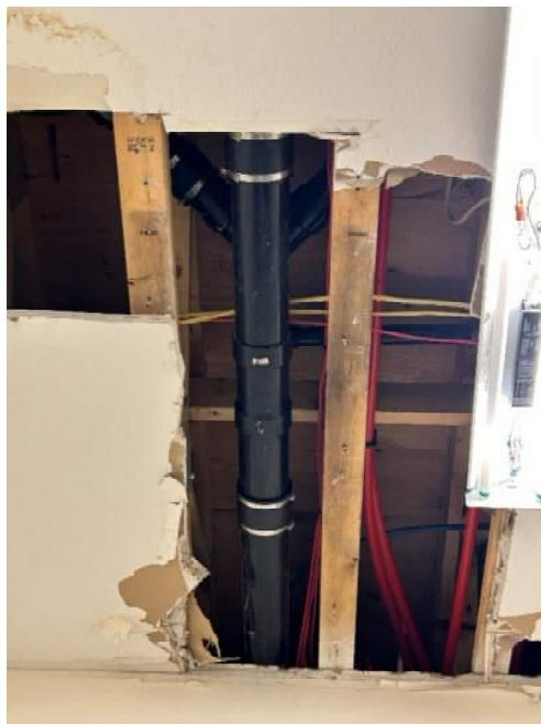
Photo 3: Exposed Main Floor Framing
