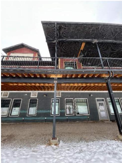
**Photo 7: Exterior Balcony – West View, with Observed Differential Elevations**
