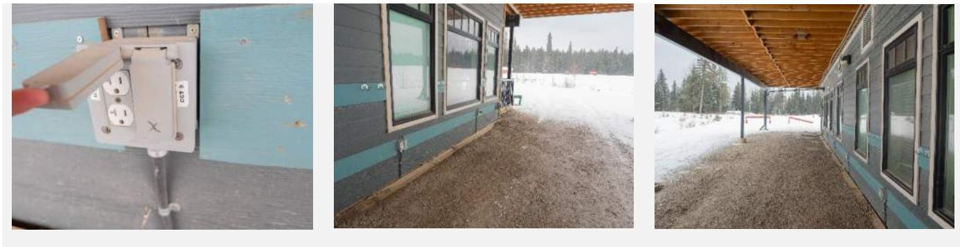
Receptacles on the balcony level are provided with cover plates, but these are not wet location extra duty covers as required by CEC. To meet the current edition of the CEC, these receptacles must be equipped with code-compliant covers.
